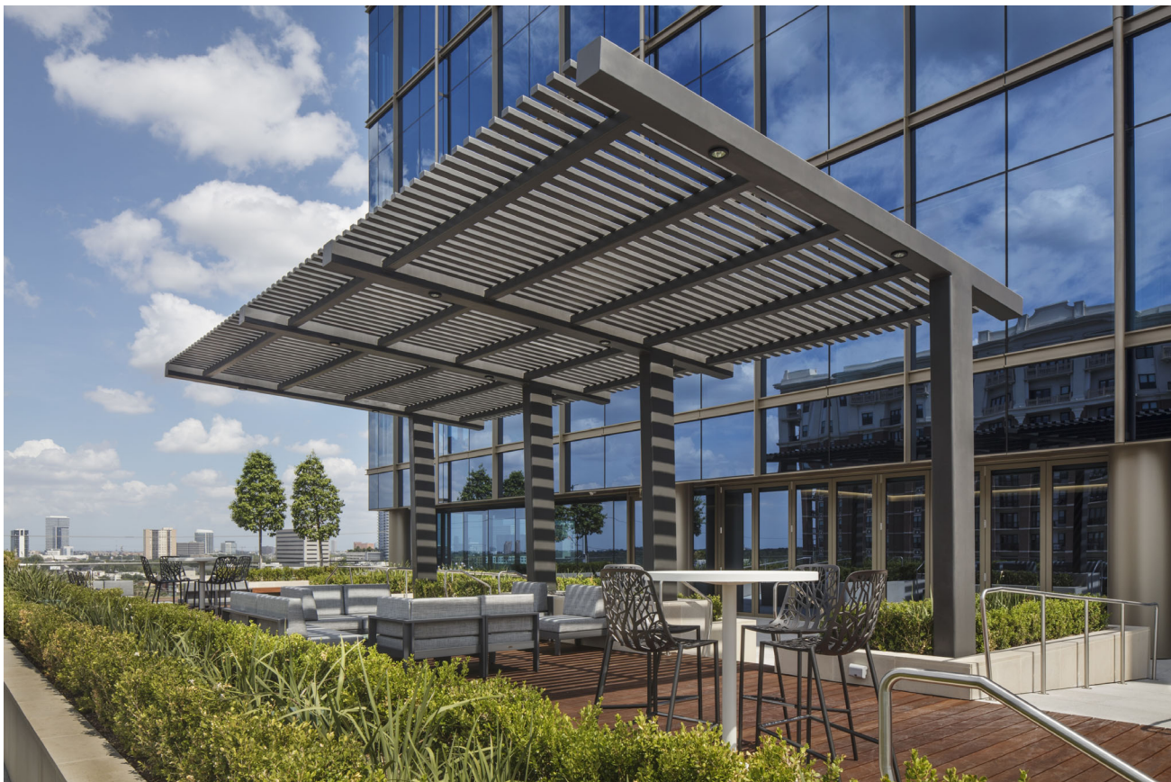
An outdoor terrace and meeting area at 200 Park Place. (Stonelake)
