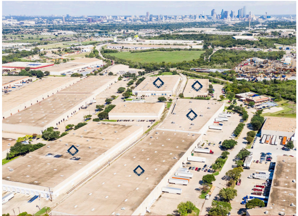
A majority of the local portfolio sold are buildings located in West Dallas.
