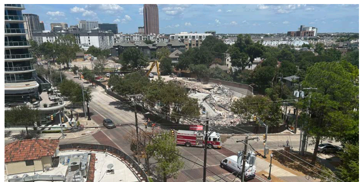
The older office building at the northeast corner of McKinney Avenue and Routh Street in Uptown was demolished on Aug. 15, 2024.
